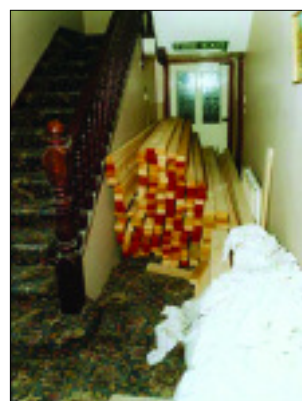
Figure 9: A blocked corridor with incorrect signage
