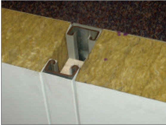
Figure 17: Insulated core panels – internal
