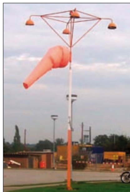
A windsock illuminated by downward-facing floodlights
