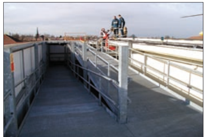
Ramp access to an elevated helipad
